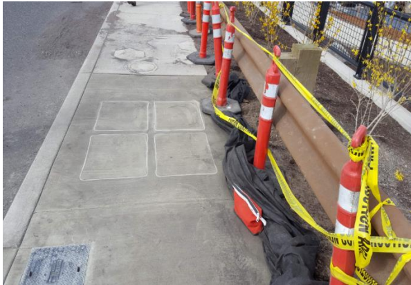
SLAB detector at Colorado Avenue in Bend MPO
